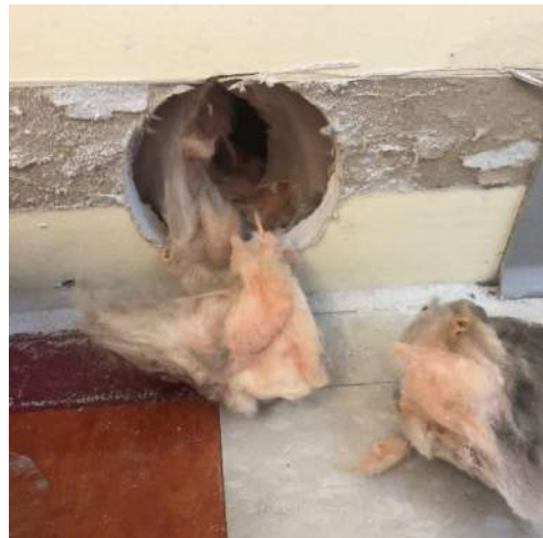
Typical condition of wall cavity batt insulation.
